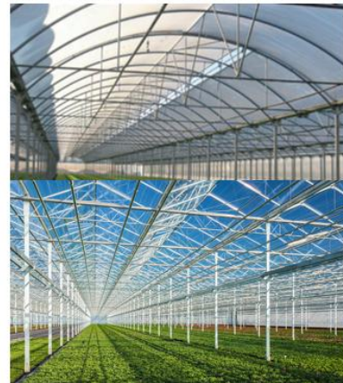
Multi-spans (multiple thermal screens)
